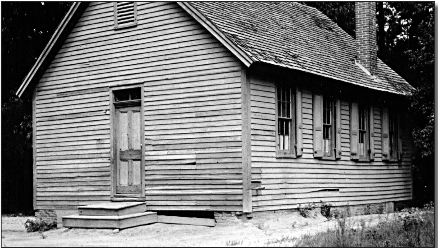
Cedar Neck White School, Sussex County, Before Renovations
