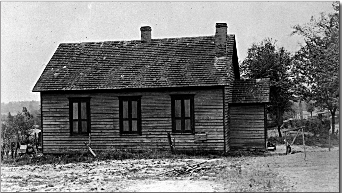
Christiana School, New Castle County, Before Renovations
