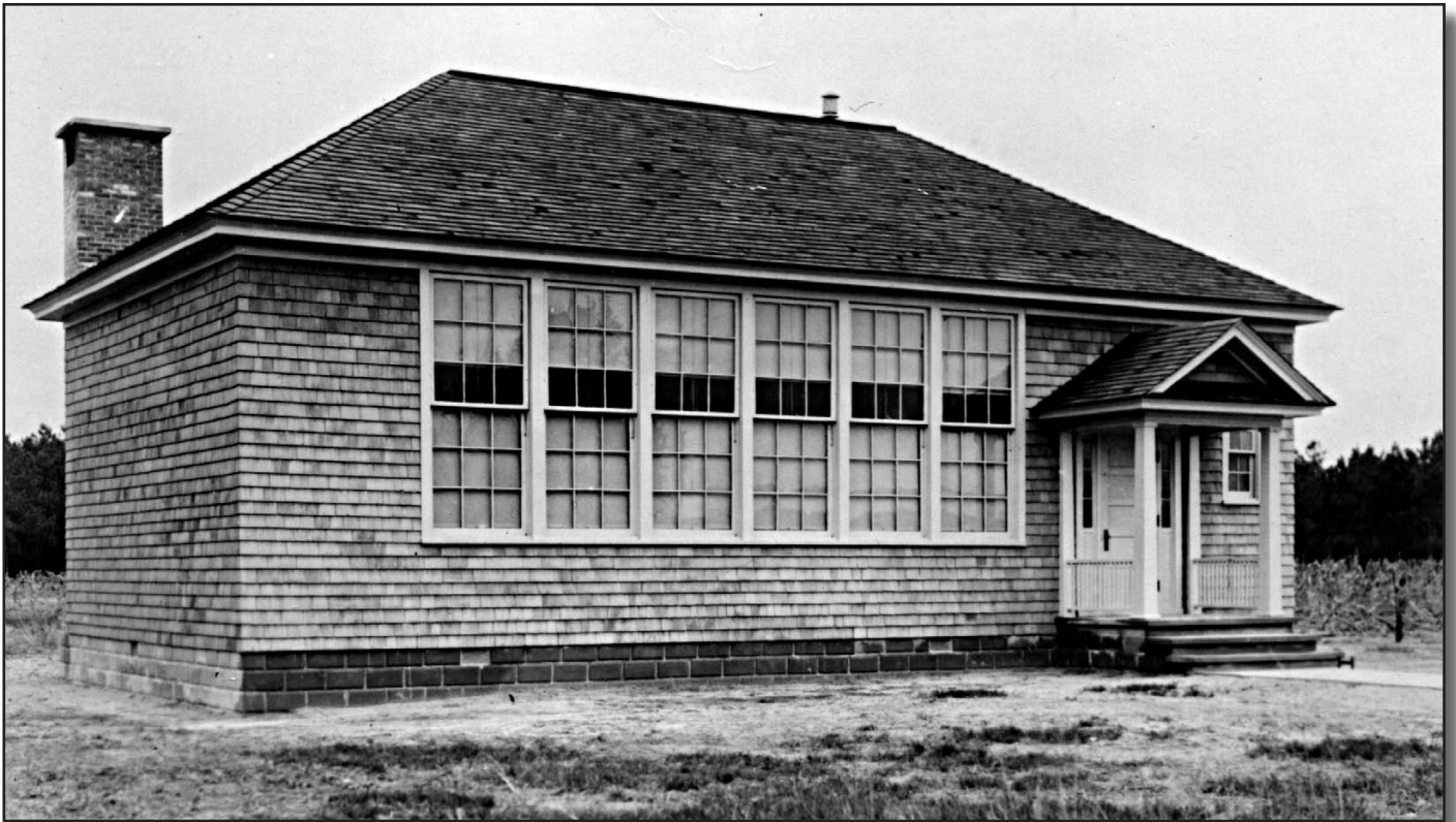
Blackwater School, Sussex County, After Renovations
