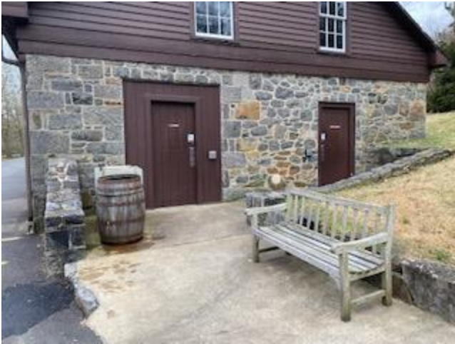
#12 Wheelwright Building – Outside Bathrooms
