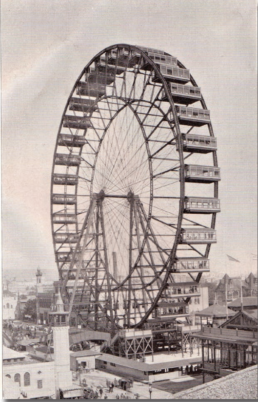
The Ferris Wheel, an engineering marvel, was constructed and first used at the World's Columbian Exposition of 1893. It was designed to rival the Eiffel Tower offered by the French at the 1889 fair. The wheel took twenty minutes per revolution with thirty-six cars holding sixty passengers each.
